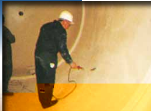
Ready in 72 hours. Final inspection
