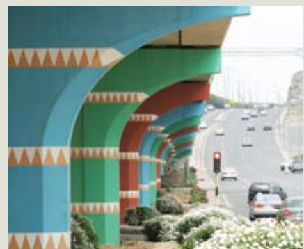
Abha Bridge, Abha, KSA
