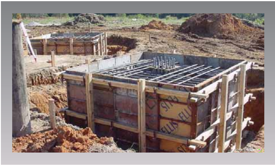
Formwork in place
