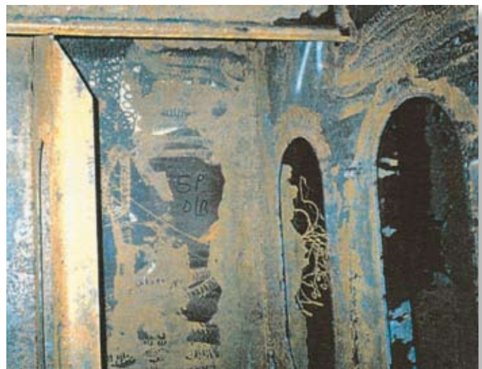
The circular effect of the waterjetting equipment leaves distinctive shapes which can be seen on the bulkhead.
