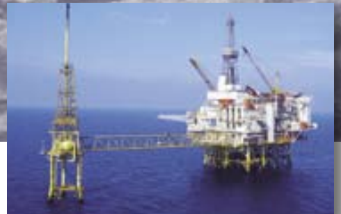
Ekofisk platforms in the North Sea – painted offshore 20 years ago with 2 x 700 microns Baltoflake. Still in very good condition without maintenance.
