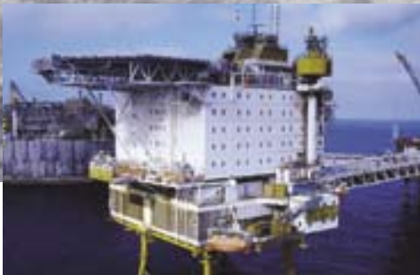
Ekofisk platforms in the North Sea – painted offshore 20 years ago with 2 x 700 microns Baltoflake. Still in very good condition without maintenance.
