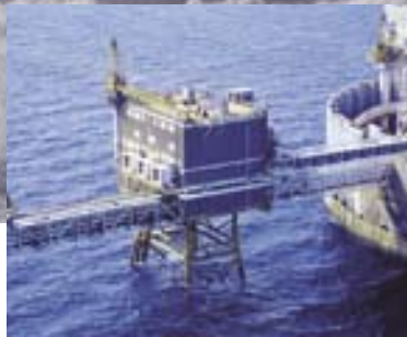
Ekofisk platforms in the North Sea – painted offshore 20 years ago with 2 x 700 microns Baltoflake. Still in very good condition without maintenance.
