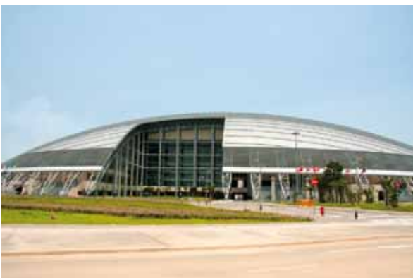
Macau Dome, Macau, China
